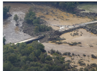
Damaged Bridge & Flooding due to Hurricane Helene, Nolichucky River, Greene County, TN, 2024 –Image courtesy of AP Photos/George Walker IV
