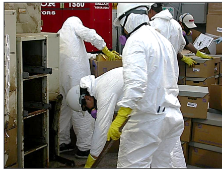
Photo courtesy of NARA—New Orleans— post-Hurricane Katrina 2005—Contractor response
